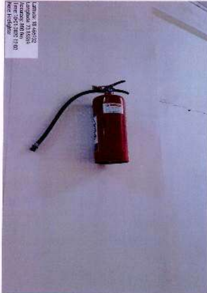
Fire extinguisher installed at institute
