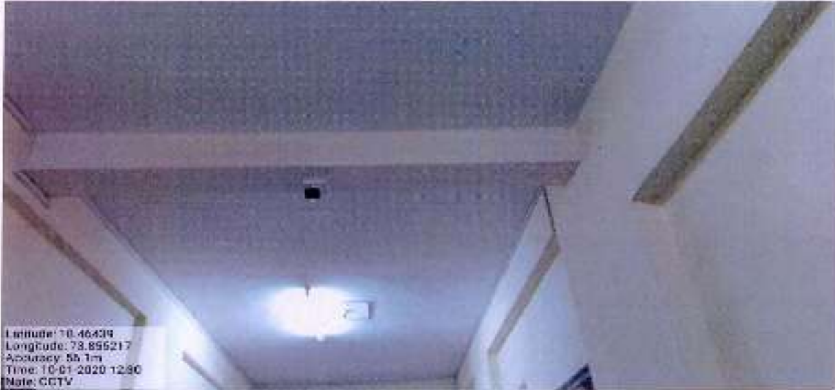
CCTV Installed in Corridor
