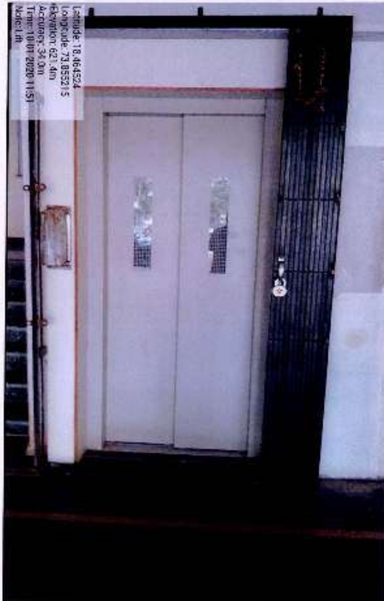
Lift facility in institute
