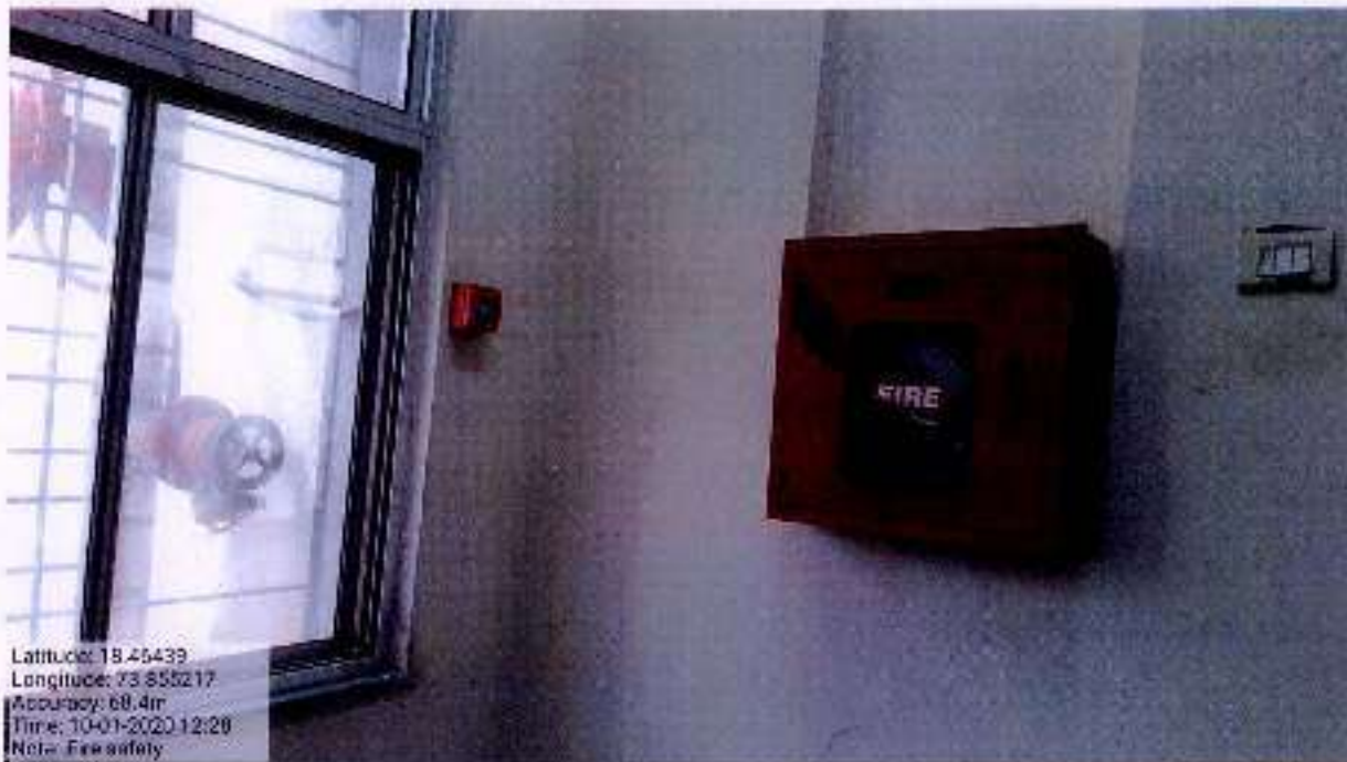
Fire safety device installed at institute
