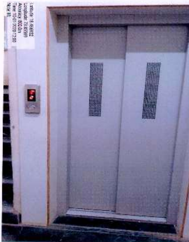
Lift facility in institute
