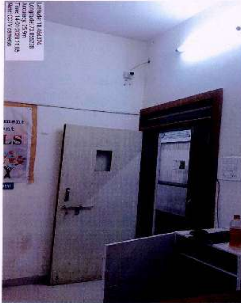
CCTV installed in classroom
